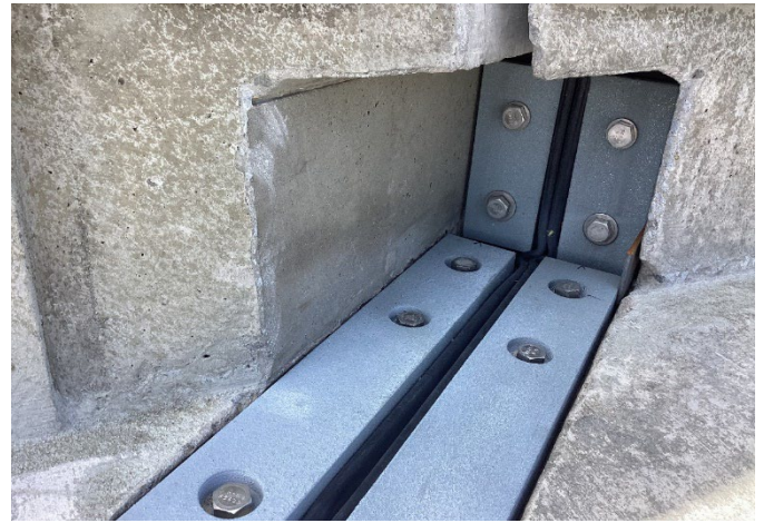
FIGURE 1 - METALLIZED EXPANSION JOINT SEAL
